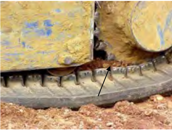
Untracking due to gravel in roller path
